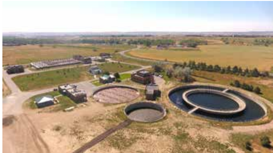
Figure 2 - City of Louisville Wastewater Treatment Plant
