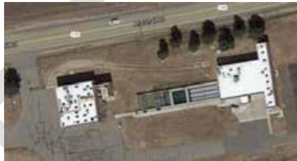
Figure 4 – Aerial View of the HBWTP
