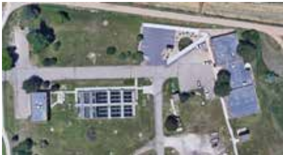
Figure 3 - Aerial View of the SCWTP
