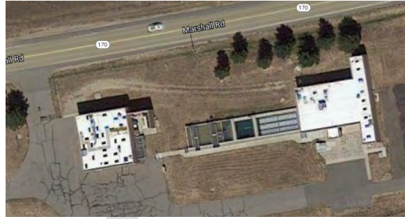
Figure 4 - Aerial of the HBWTF
