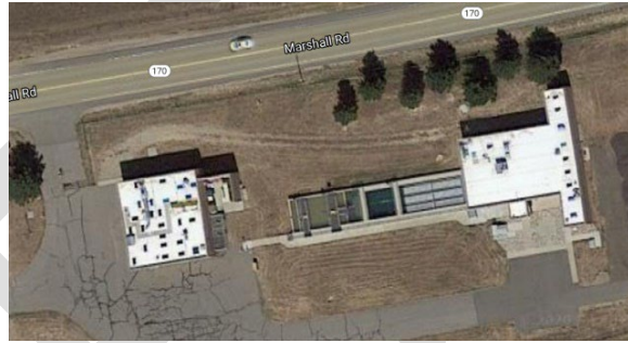
Figure 4 – Aerial View of the HBWTP
