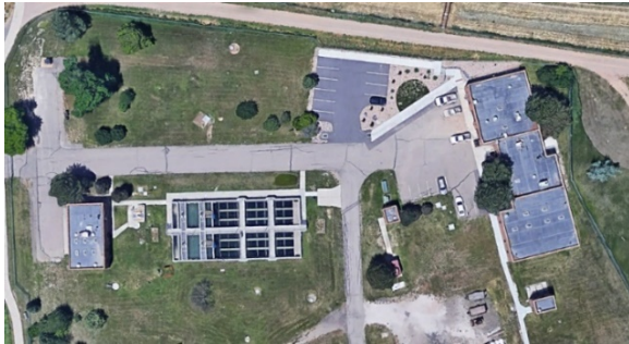
Figure 3 - Aerial View of the SCWTP
